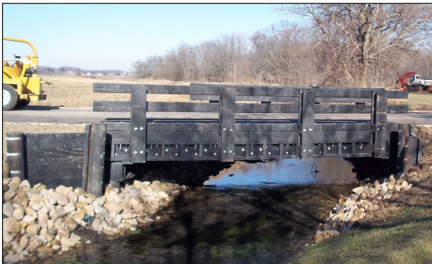
Bridge 174-0.56 over the Onion Ditch
